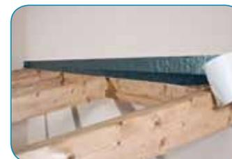
Begin the project by installing the flashing tape to provide a watertight seal between the wall and roof.
